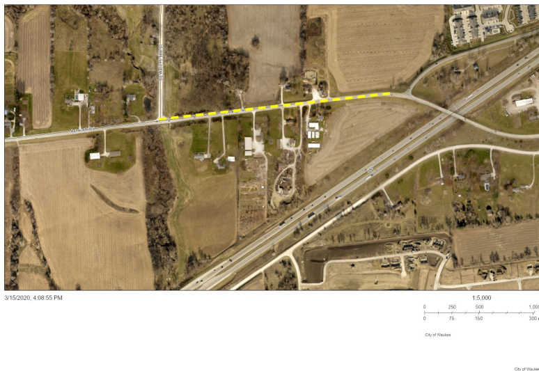
Ashworth Rd Reconstruction - WDM Project
