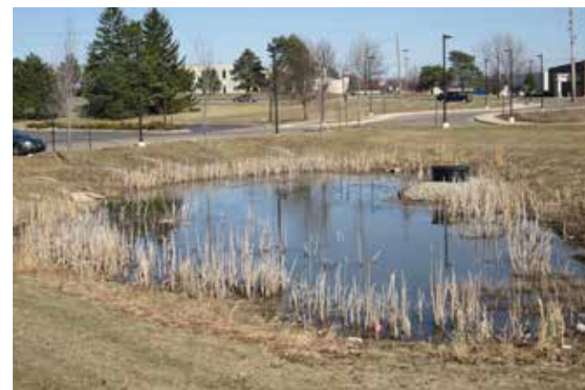
Example of a small detention basin. This type of detention is discouraged within Kettlestone.
